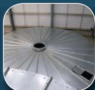
Flat Roof Silos
